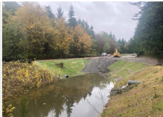
Photo 2: Greenwood Pond – Looking SE
