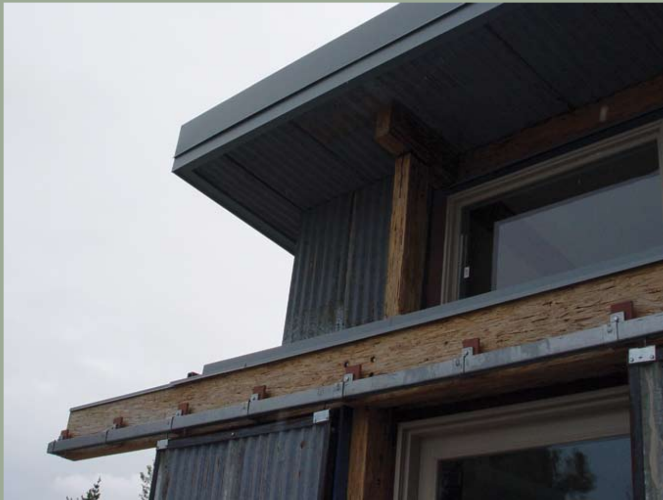
Washington State University - Zero Energy House, Shoreline Community College Campus
